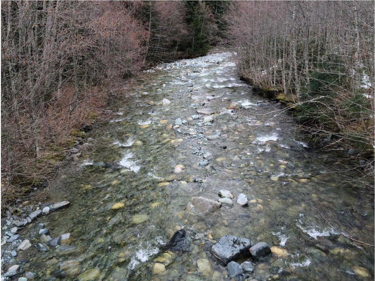
Photograph 11. On Bridge over Raley Creek, looking east (Lat: 54.180692, Long: -128.682419)
