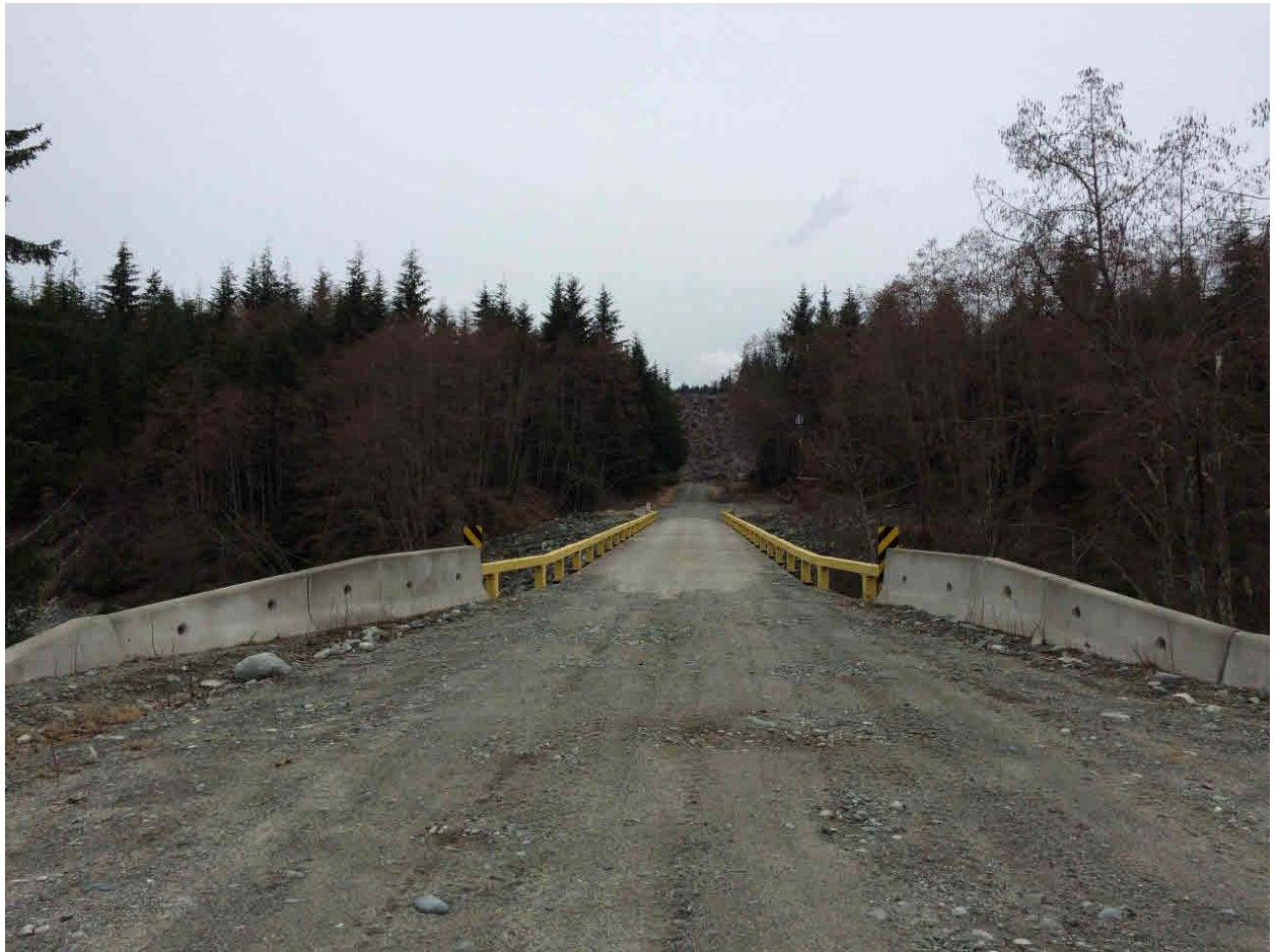
Photograph 7. Bridge #4 along Wedeene FSR, looking north (Lat: 54.13508, Long: -128.68301)
