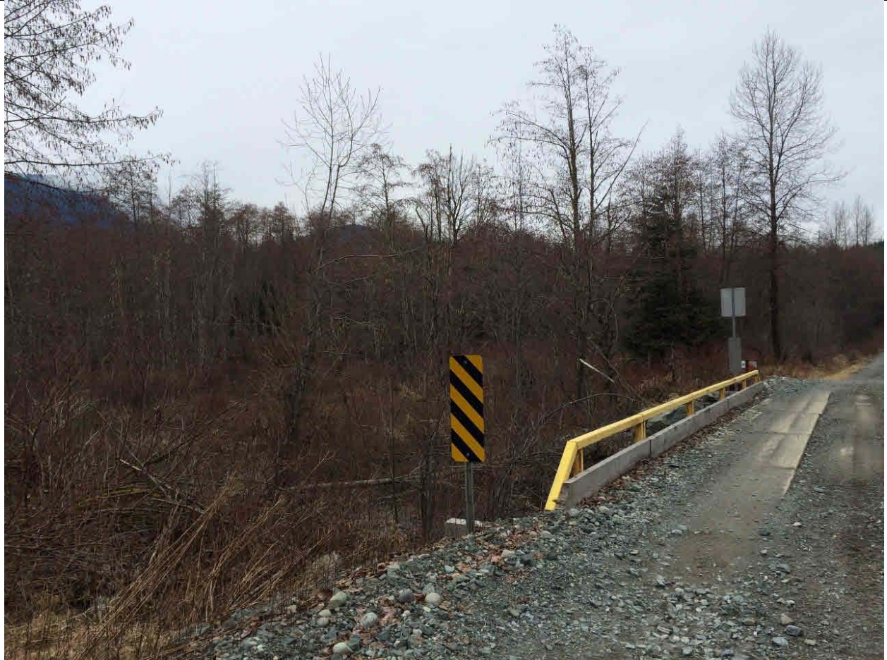
Photograph 3. Bridge #2 along Wedeene FSR, looking north (Lat: 54.08105, Long: -128.67713)
