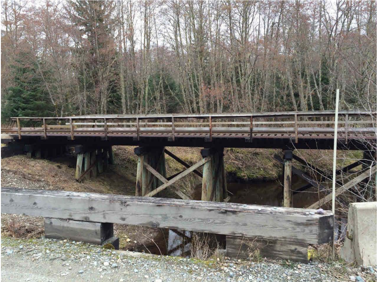
Photograph 6. Bridge #3 along Wedeene FSR, looking east towards CN Main Rail Line (Lat: 54.08105, Long:- 128.67713)
