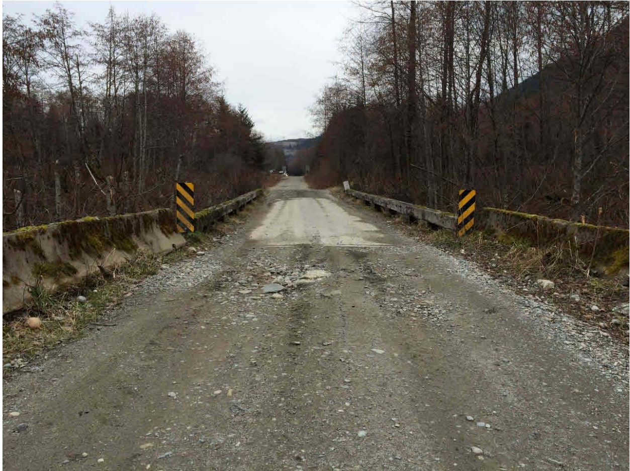
Photograph 2. Bridge #1 along Wedeene FSR, looking north (Lat: 54.068068, Long: -128.690373)
