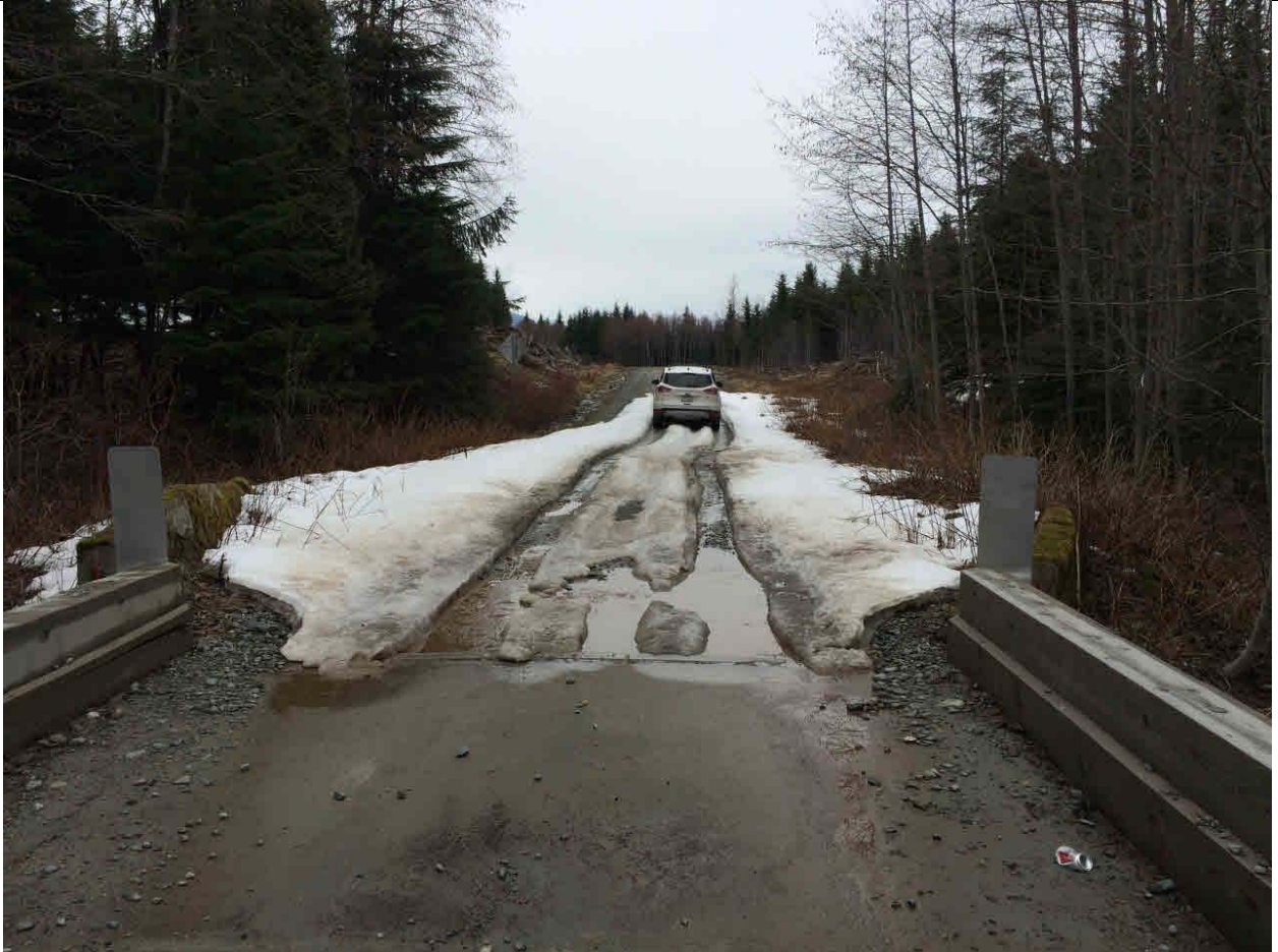
Photograph 10. Bridge #5 along Wedeene FSR, looking north (Lat: 54.14962, Long: -128.68553)
