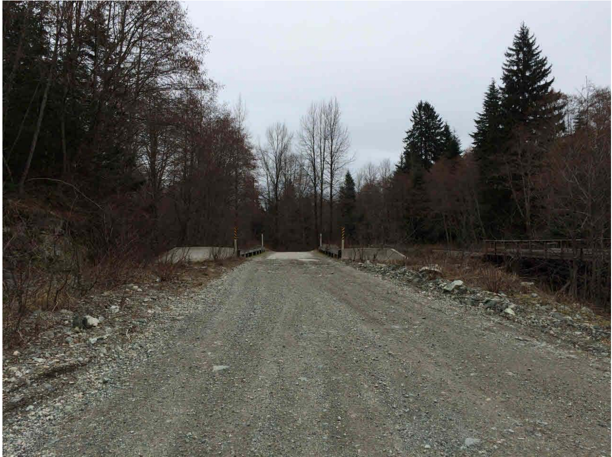
Photograph 5. Bridge #3 along Wedeene FSR, looking north (Lat: 54.08105, Long:- 128.67713)
